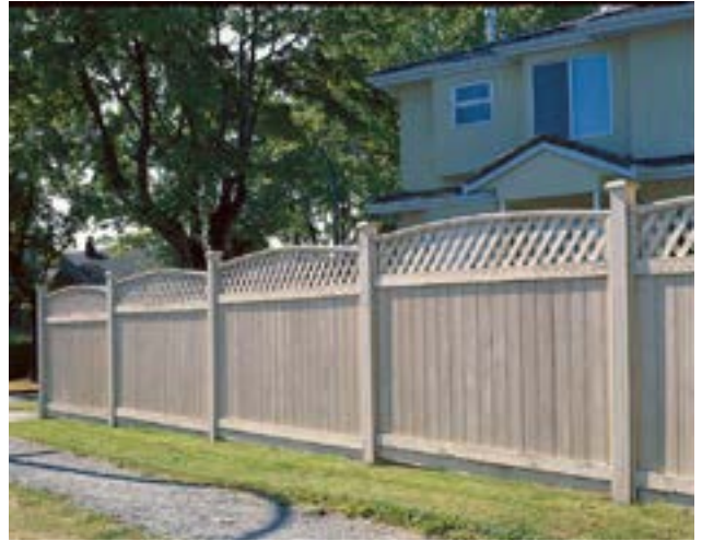
The graceful curve of the top rail and latticework reduce the scale of this solid board fence.
