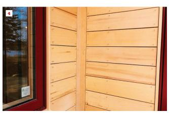
Siding nails directly over commercially available rainscreen materials like this mesh (1). With site-built systems, the siding nails to furring strips (2). With a closed rainscreen, the siding installs with a lap joint or it overlaps, as with clapboard (3). In an open rainscreen, the siding nails to the furring strips with air gaps between the boards (4).
