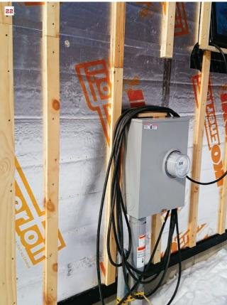
A carpenter scribes a board around a window in an open rainscreen system, with spacing between the boards and a space left under the window sill (19). A temporary strip creates the open space at a corner board (20). Furring strips end well above the head flashing over a window (21). Services such as this electrical meter are furred off the wall as part of the siding (22).
