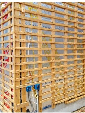
A second horizontal layer of furring provides nailing for vertically applied siding, such as this corrugated metal (10). If there isn't enough depth for the second layer of furring, the strips can be installed diagonally with breaks to allow water to drain down and out of the bottom (11). Site-built rainscreens can be used for shingle siding, but this application is labor intensive (12).
