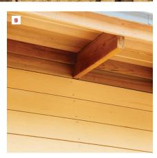
Site-built rainscreens install over the WRB, so it should be complete with all seams and openings sealed and flashed properly (5). With an open rainscreen, building paper covers the WRB to protect it from UV rays (6). Protection from critter intrusion can be either mesh (7) or corrugated vent material (8). Air space at the top of the wall allows ventilation for drying (9).
