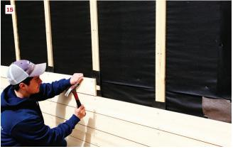
Open rainscreen systems leave the furring strips exposed in the gaps between the boards. Many different strategies can be employed to hide the natural color of the strips. One option is painting the strips before they go on (13). The entire furring strip can be covered with building paper (14), or tabs of building paper can be inserted as the siding goes on (15).
