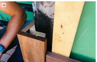
Seal all window openings and integrate them with the WRB. A flap of building paper below the window (16) layers into the building paper of the open rainscreen so that it sheds water properly (17). This mock-up of a corner shows how to leave the boards open for maximum air circulation in an open rainscreen system (18).
